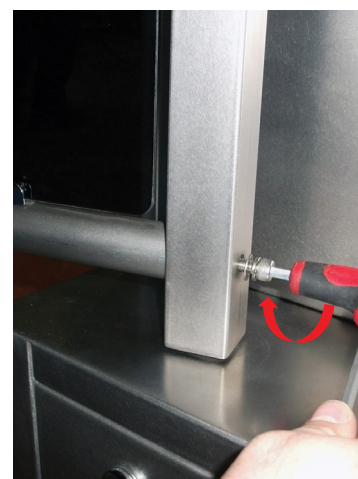
3. Tighten bottom fixing screw
